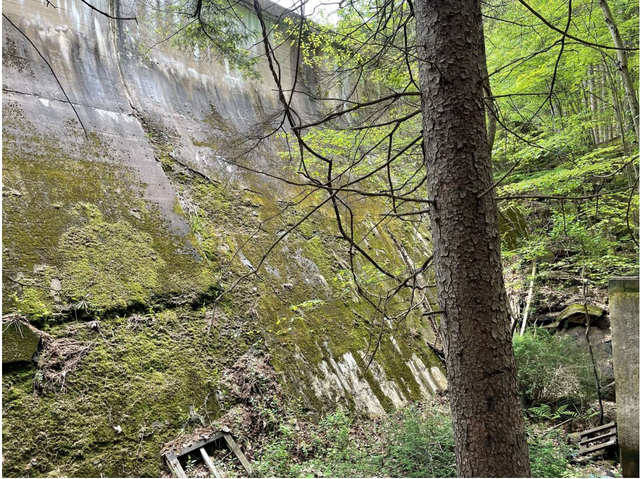
Photo 3 – Hackettstown Reservoir Downstream Face – Musconetcong Watershed Association - 2024
