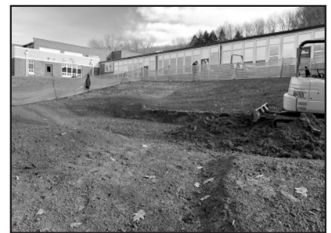
Rain Garden at Hoppock Middle School, under construction
