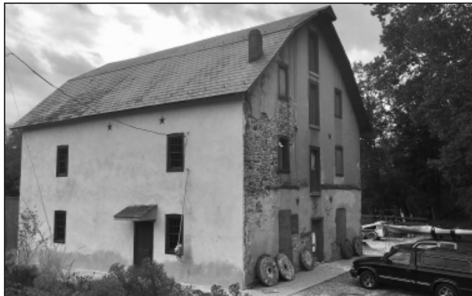
Asbury Mill East wall with new stucco
