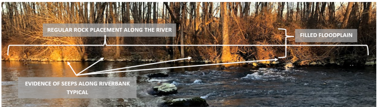
Figure 7: View of south/east bank of the Musconetcong River toward the western area of the Haberman Hampton Tract. Note regular stone placement and filled floodplain and note exposed limestone boulders in river in the foreground. Date: January 17, 2020.
