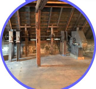
We made significant progress on the Asbury Mill in 2016. The main accomplishment was completing all of the structural repairs in the interior of the building. This included replacing: all of the broken or damaged floor joists on the first, second and third floors; support columns where necessary and flooring throughout most of the building—including installing a new basement floor with radiant heat.
