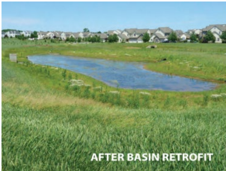
Figure P.8 – 24 hours after a storm and the stormwater is spread out and native vegetation is allowing the water to naturally infiltrate and recharge the groundwater, instead of being piped to surface water streams. Images - https://pecpa.org/
