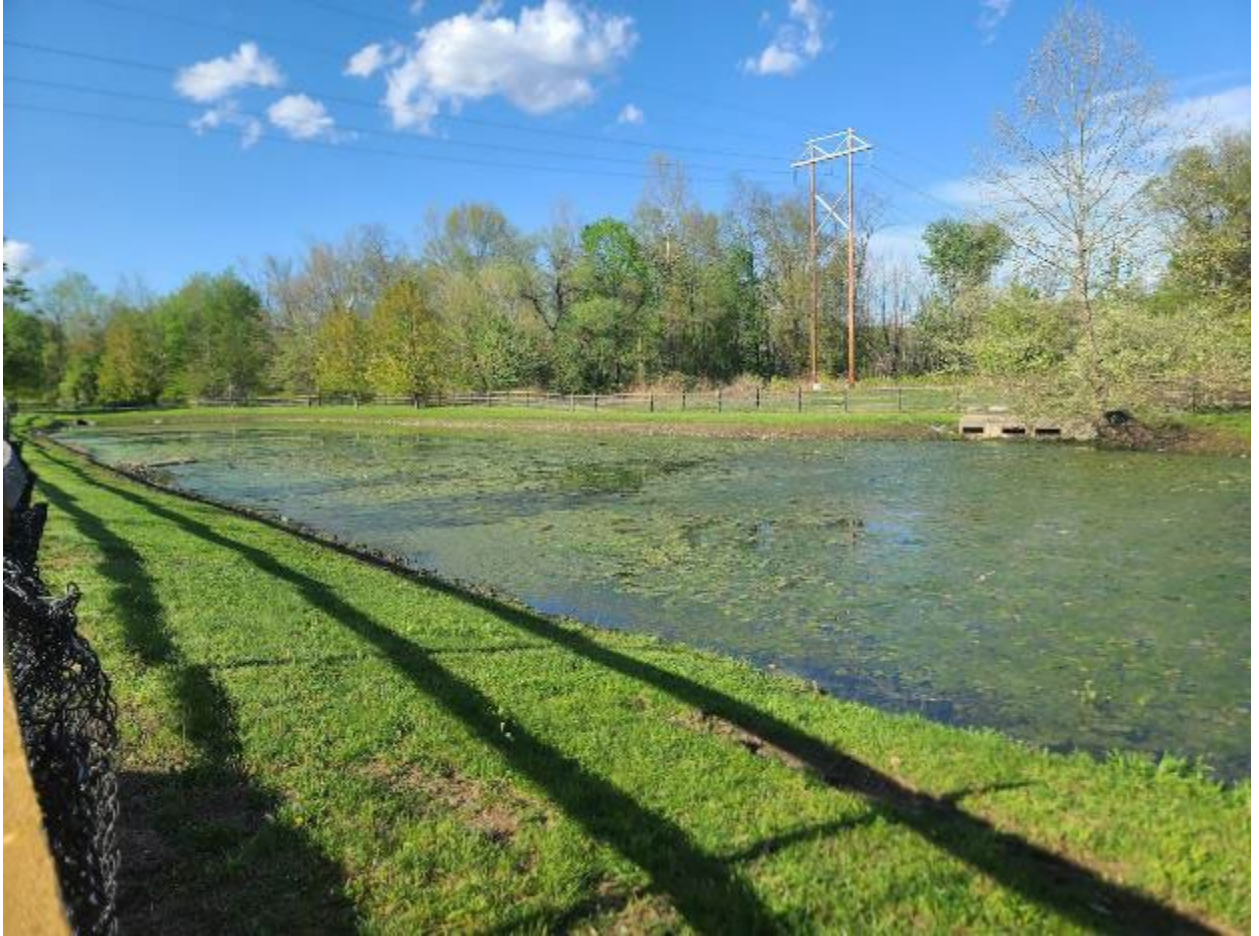
Figure P.4 – Wet detention basin in Hackettstown NJ. This basin is overrun by algae and has many Canada Geese in residence (not in picture). It drains directly into the mainstem of the Musconetcong River. Photo Credit – MWA
