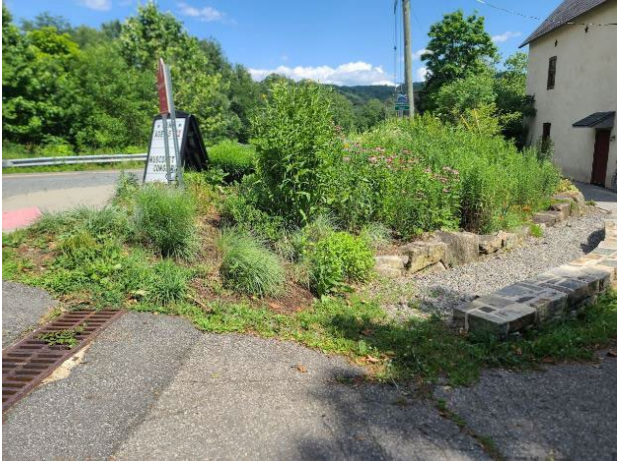
Figure P.2 -Rain Garden on Main Street in Asbury, NJ. A trench captures runoff and pipes it into the rain garden. Photo credit – MWA
