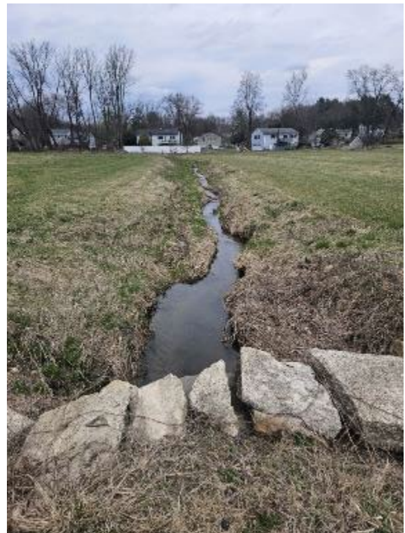
Figure B: Showcases the right branch flowing from the residential neighborhood and through the agricultural pastureland and the lack of stormwater infrastructure on the way.
